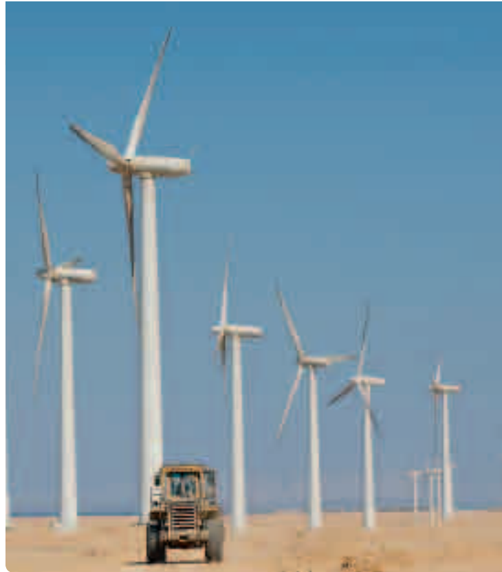
Zafarana wind farm, Egypt
