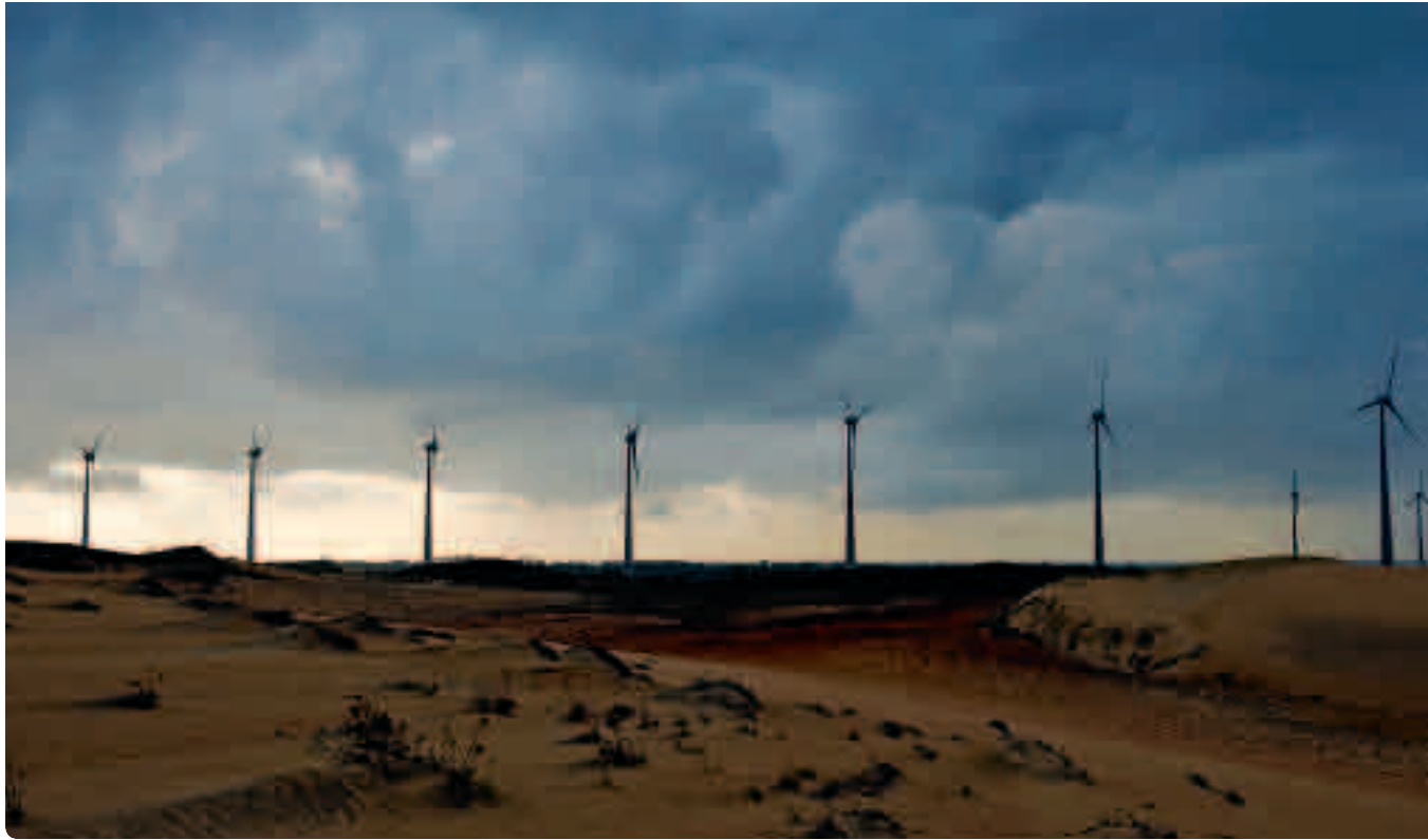
Rio do Fogo wind farm, Brazil © Wind Power Works
