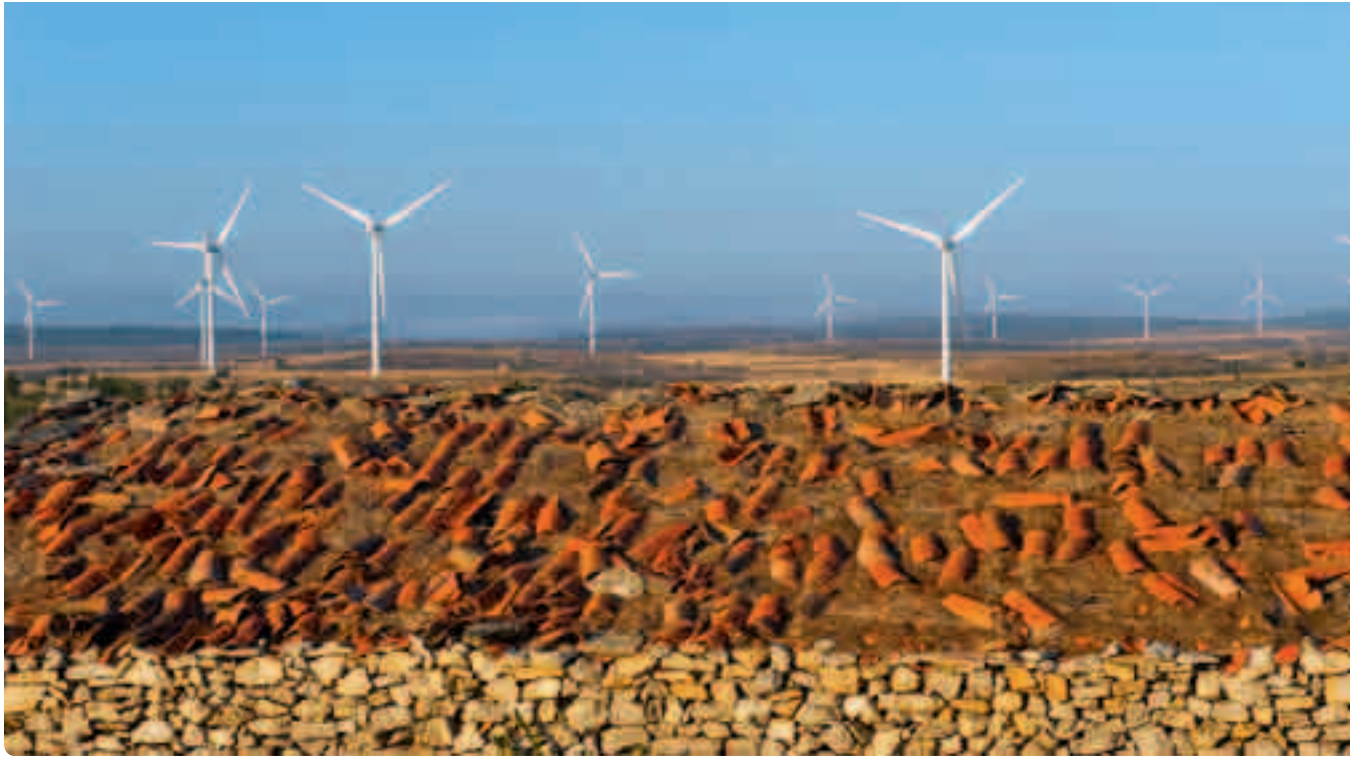
Maranchón wind farm, Guadalajara, Spain © Wind Power Works
